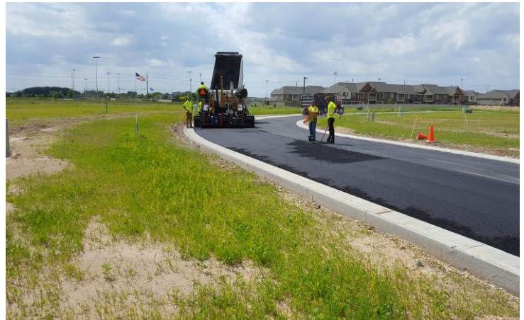
Crosswind Estates Paving
